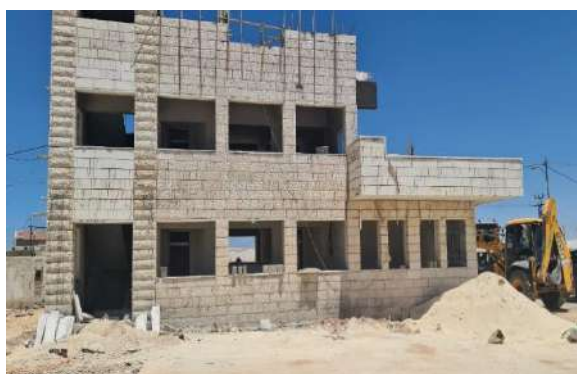
Construction of buildings
