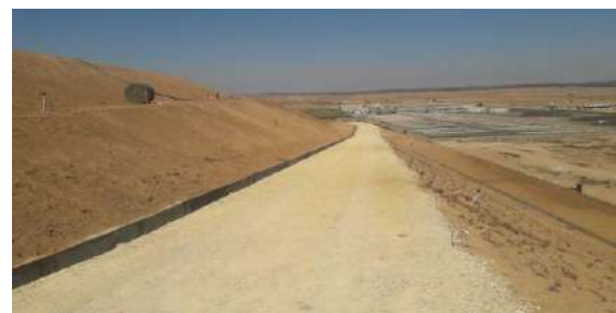
Final Covering System at Al-Fukhari (Sofa) dumpsite
