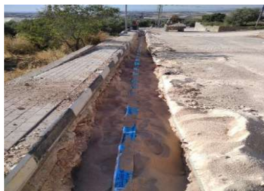
Construction of water distribution network
