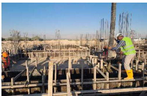
Casting concrete for poultry building
