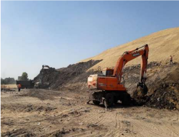
Reshaping and Covering operations of Dair Al Balah Landfill
