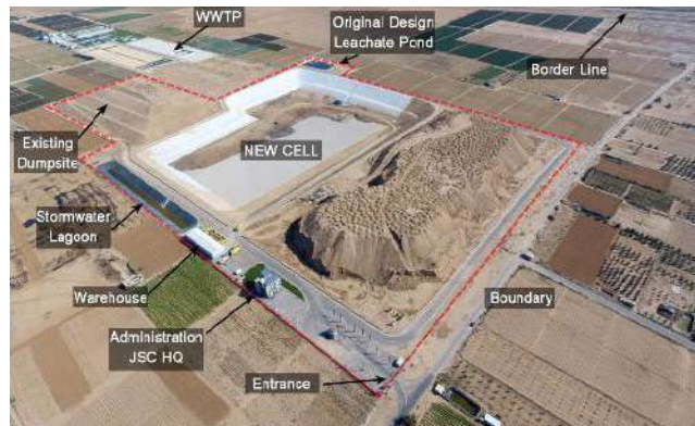
Al-Fukhari Sanitary Landfill and Surrounding Area
