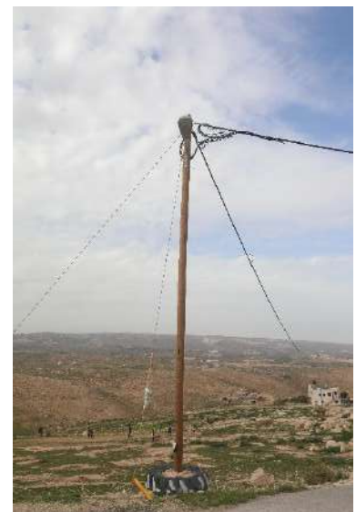
Om Adaraj - Al Ka'abneh. Rehabilitation of the Electrical Network
