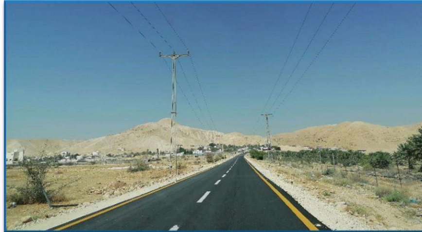
Municipal Garage road
