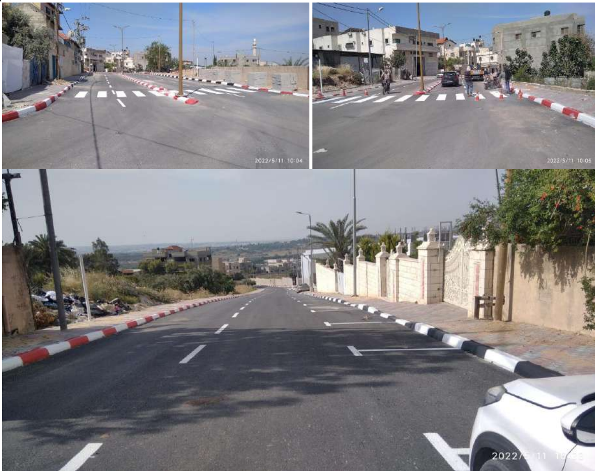
Rehabilitation of an Internal Road
