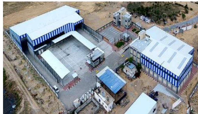
Rafah Transfer Station Compound
